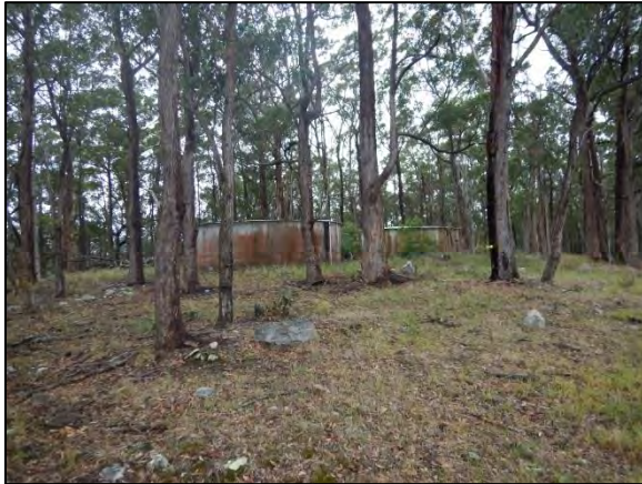
Figure 8: View of existing water tanks at eastern extent of Stage 2
